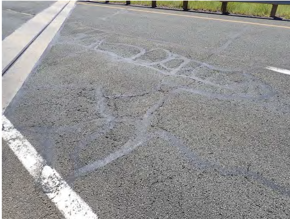
Photo 8: Transverse Crack in Asphalt, Eastbound at Milepost 51.4
