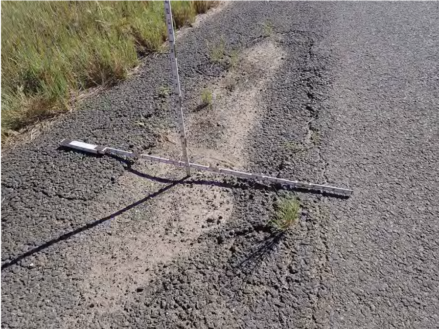
Photo 2: Overall of Rutting in North Shoulder, Westbound at Milepost 52.6
