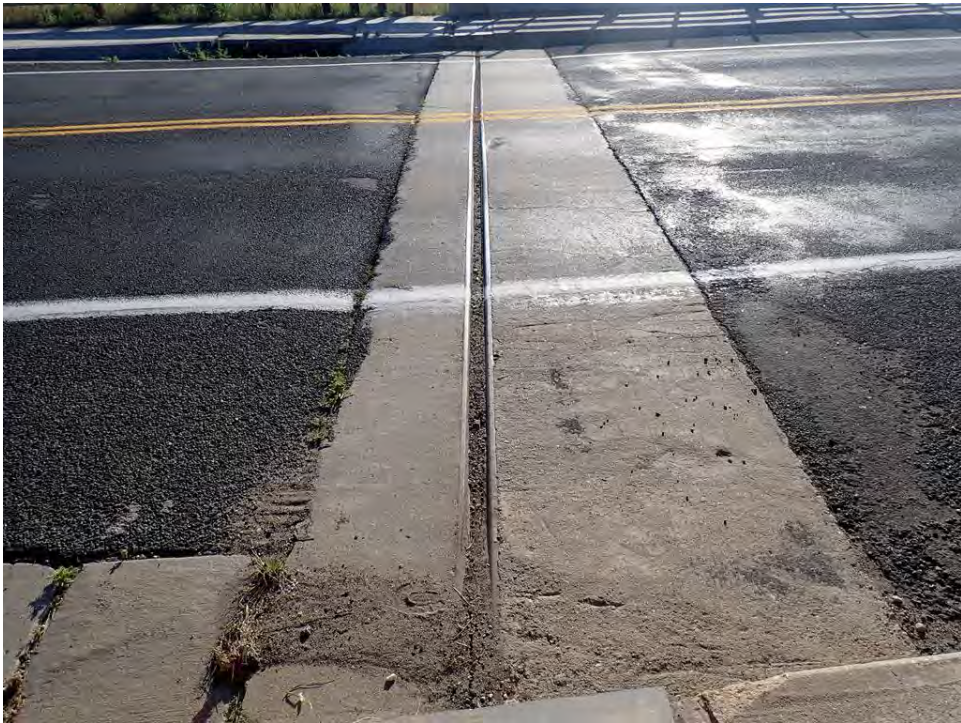
Photo 20: Dirt in Expansion Joint at 120 th Overpass
