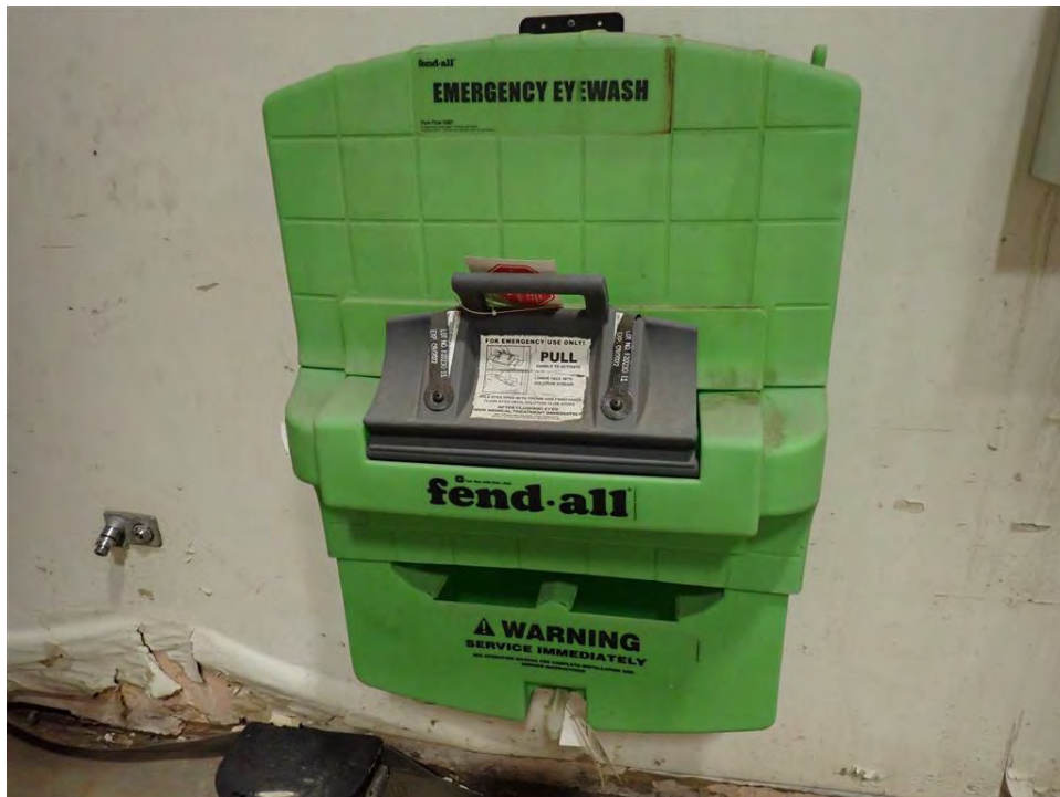
Photo 66: Eye Wash Station in Equipment Maintenance and Cleaning Building, Expired Lot Tag
