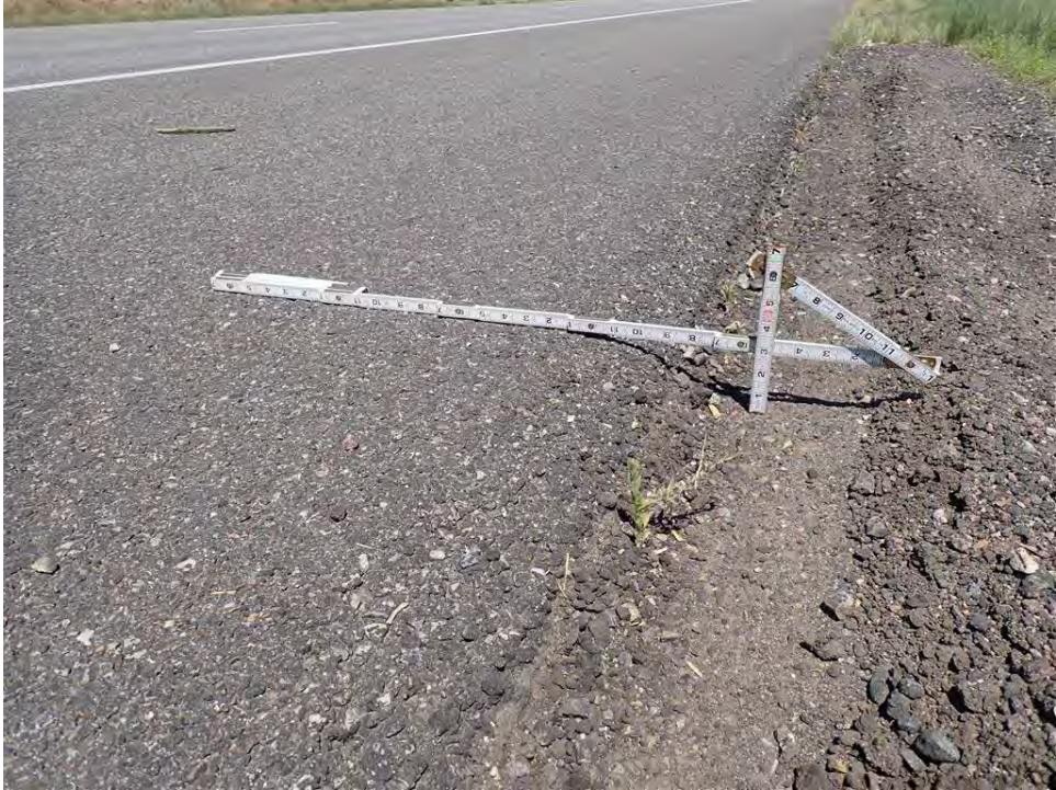
Photo 26: Shoulder Drop-Off, Eastbound at Milepost 51.15
