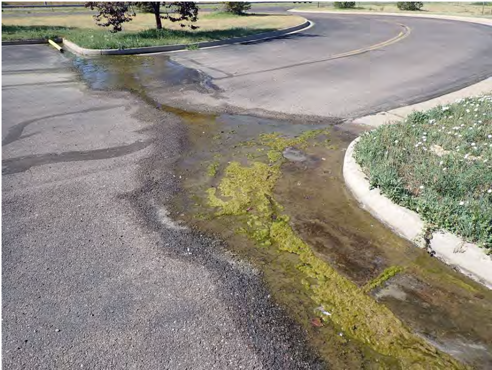
Photo 73: Drainage Across Parking Lot on West Side of Administration Building
