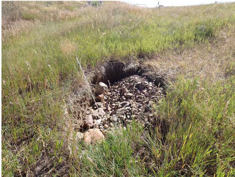
Photo 34: Erosion Trough and Displaced Riprap in North Slope, Westbound at Milepost 51.05
