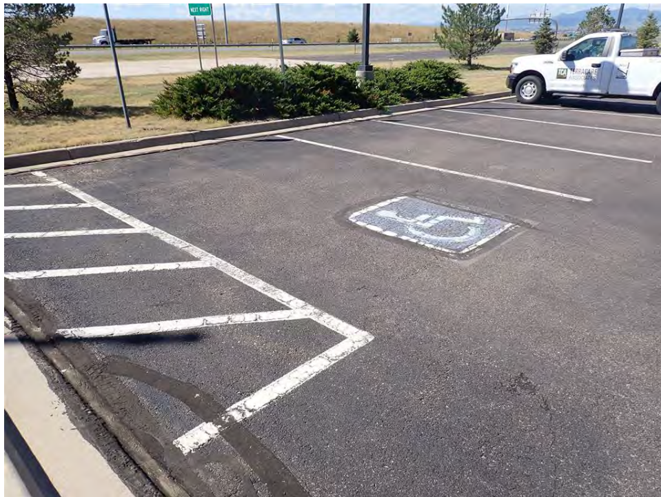
Photo 72: Faded Paint on Asphalt in Parking Lot on West Side of Administration Building
