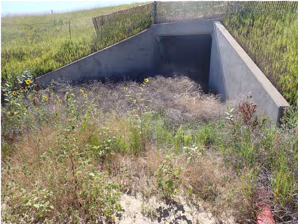
Photo 32: Erosion Trough in Median, Milepost 46.95
