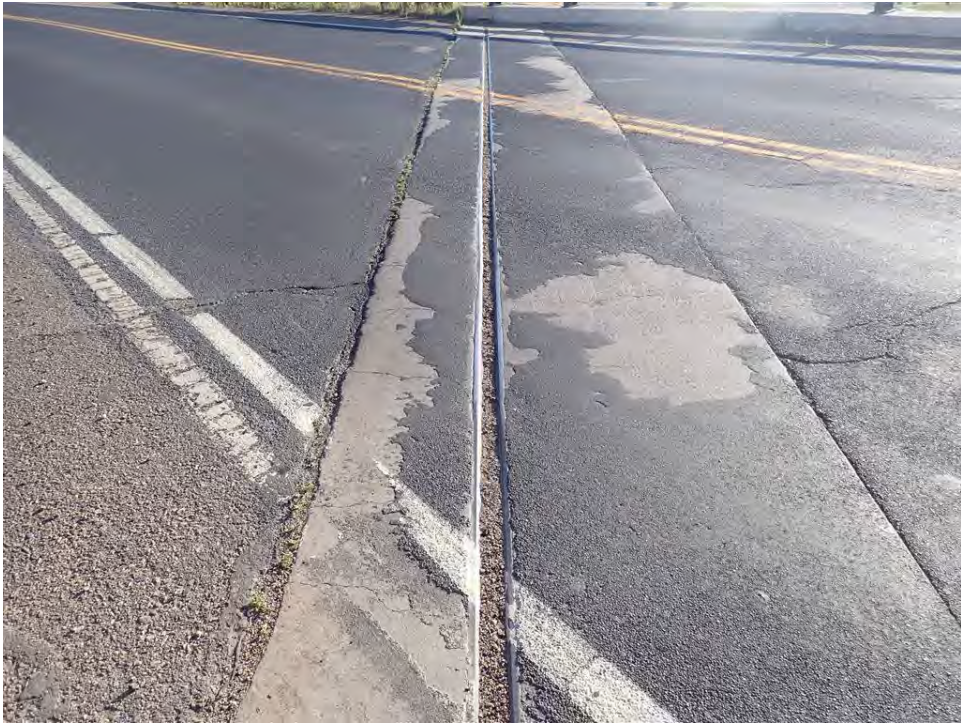
Photo 20: Dirt in Expansion Joint at 120 th Overpass
