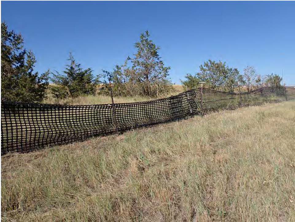
Photo 36: Loose and Sagging Snow Fence, Eastbound at Milepost 46.7
