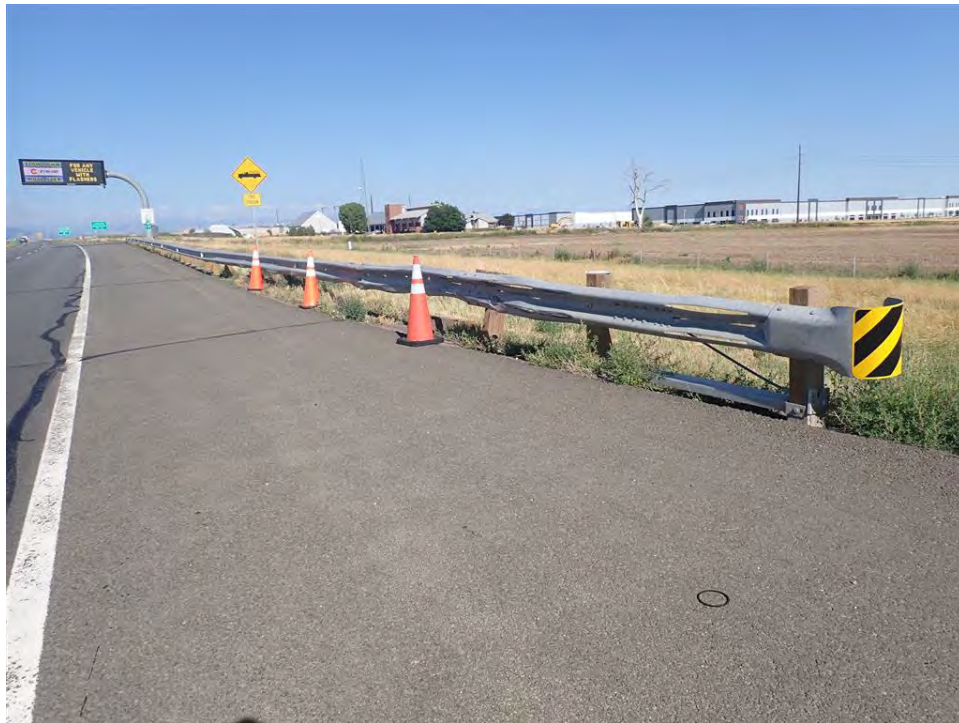
Photo 46: Impact Damage to Guardrail, Westbound at Milepost 47.35
