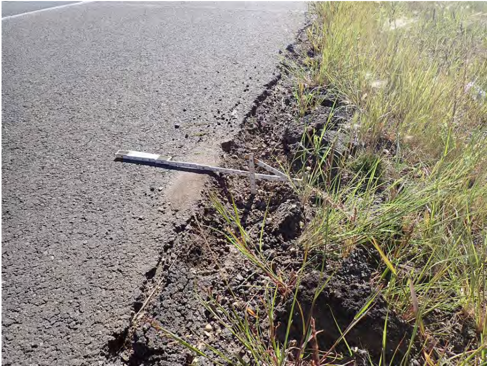
Photo 28: Shoulder Drop-Off, Eastbound at Milepost 46.75
