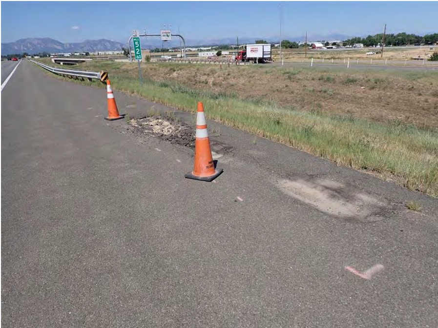
Photo 2: Overall of Rutting in North Shoulder, Westbound at Milepost 52.6
