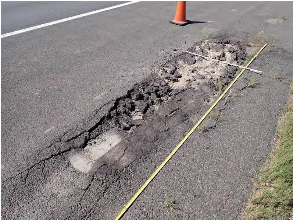
Photo 4: Asphalt Heaved up to 5 Inches at Rutting in North Shoulder, Westbound at Milepost 52.6
