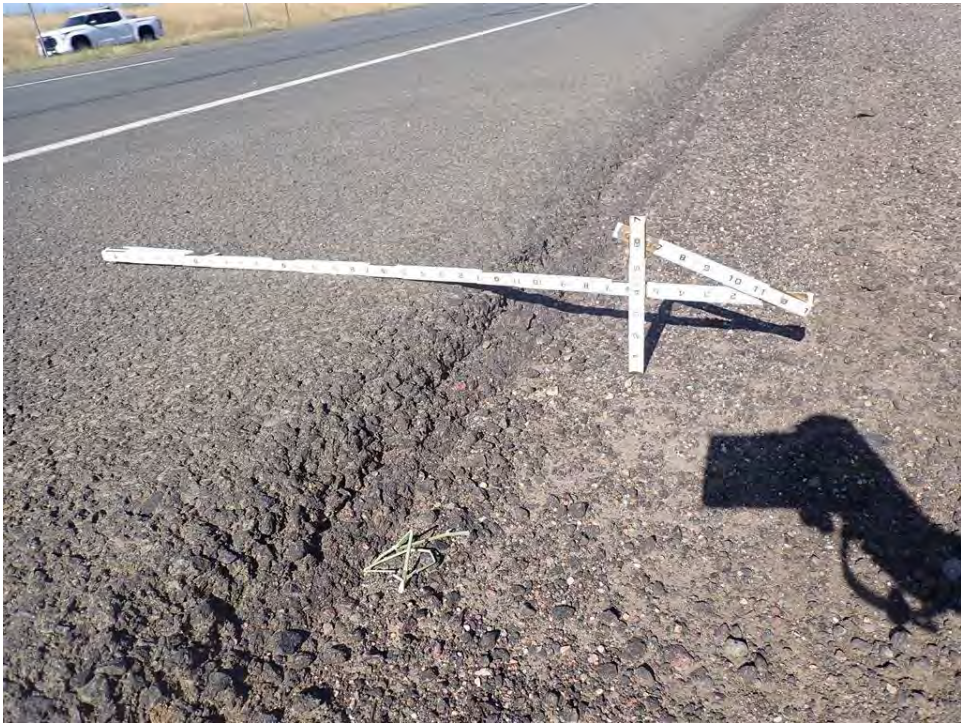
Photo 28: Shoulder Drop-Off, Eastbound at Milepost 46.75
