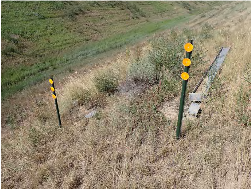
Photo 42: Sign Posts Laying in Right-of-Way, Westbound On-Ramp at US 287
