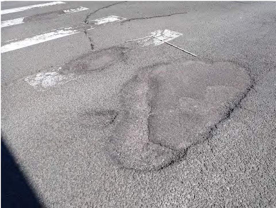
Photo 16: Repaired Potholes in Asphalt, Eastbound at 96 th Steet
