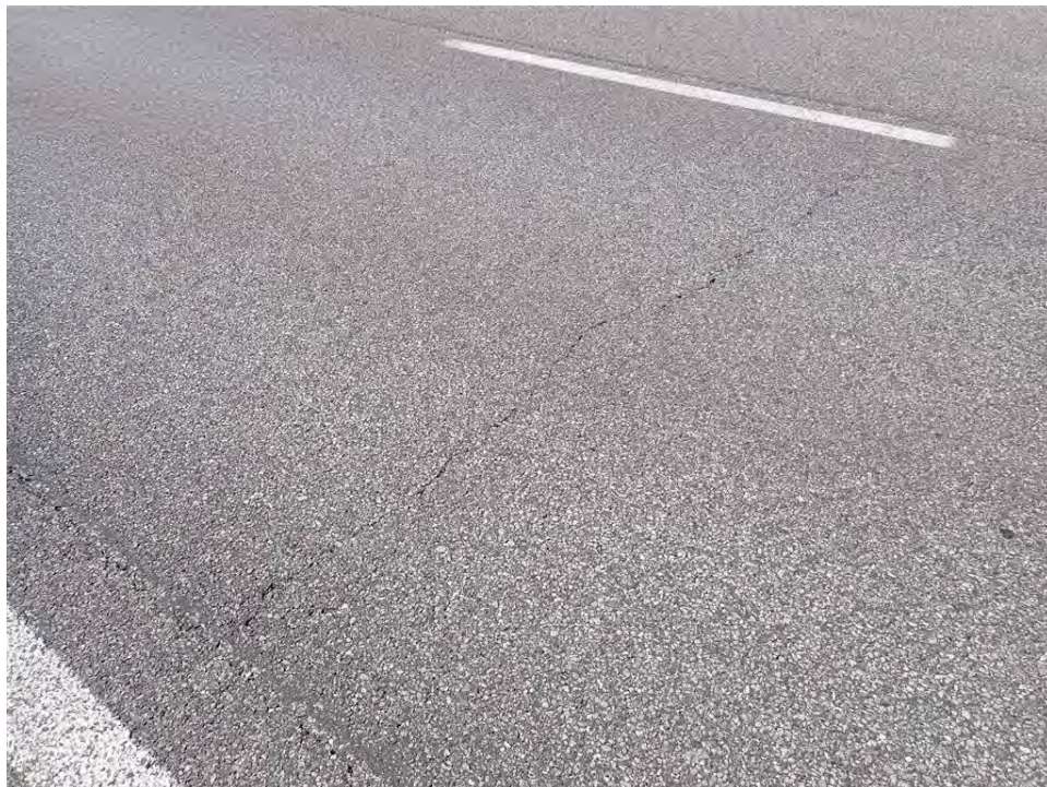
Photo 8: Transverse Crack in Asphalt, Eastbound at Milepost 51.4
