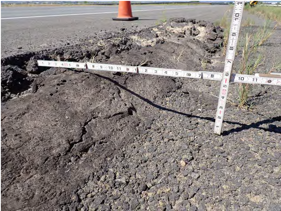
Photo 4: Asphalt Heaved up to 5 Inches at Rutting in North Shoulder, Westbound at Milepost 52.6
