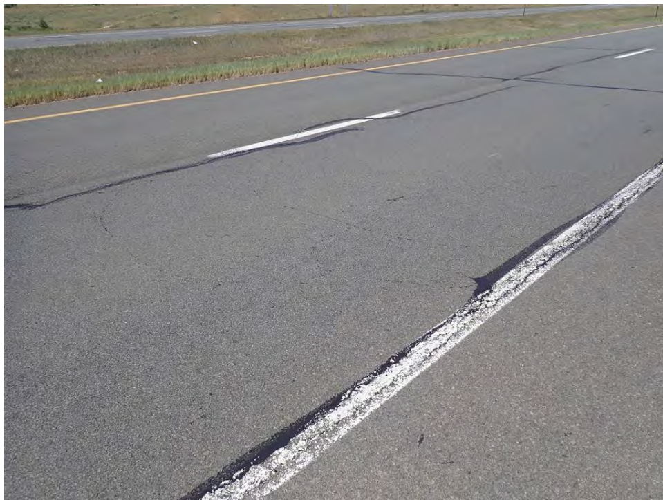
Photo 54: Typical Worn Paint (Eastbound at Milepost 51.5 Pictured)
