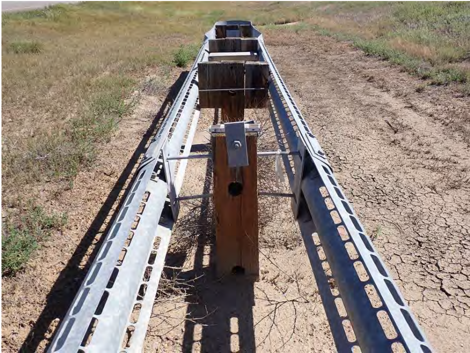
Photo 50: Typical Missing Timber Blockings in Median Guardrail (Milepost 51.05 Pictured)
