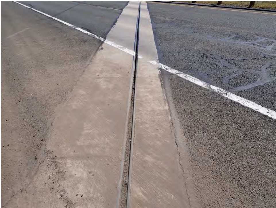
Photo 24: Dirt in Expansion Joint at Bridge over US 287, Eastbound
