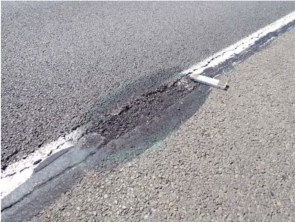
Photo 14: Patched Pothole in Asphalt, Westbound at Milepost 48.15
