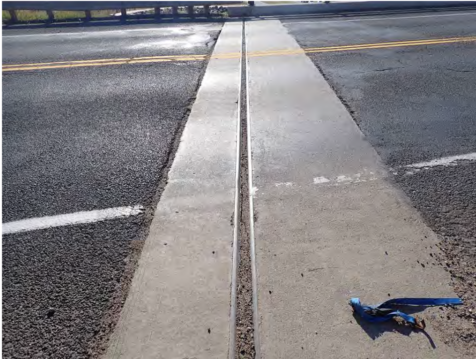
Photo 18: Dirt in Expansion Joint at Huron Overpass
