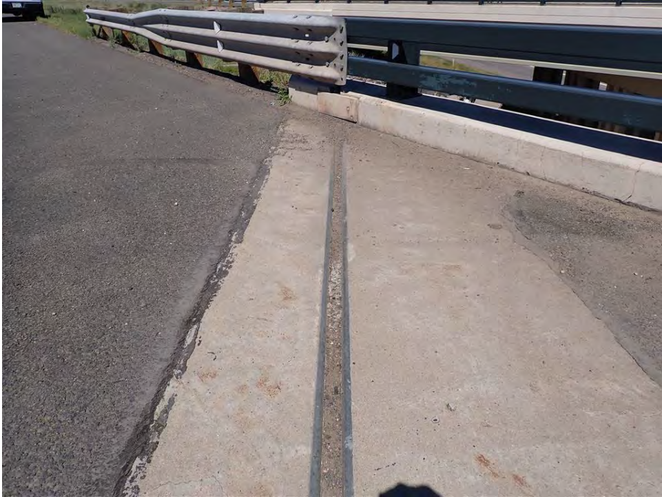
Photo 22: Dirt in Shoulder of Expansion Joint at Bridge over Eastbound Dillon Road, Westbound
