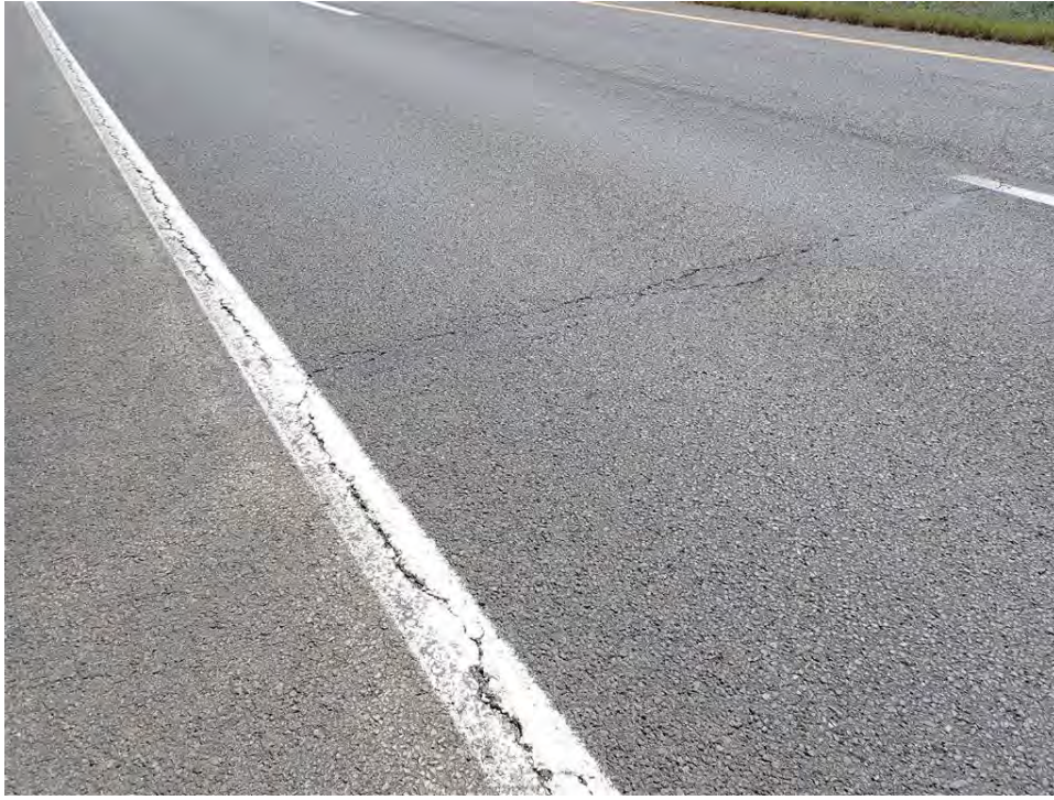
Photo 12: Poorly Sealed Longitudinal Crack in Asphalt, Westbound at Milepost 48.7
