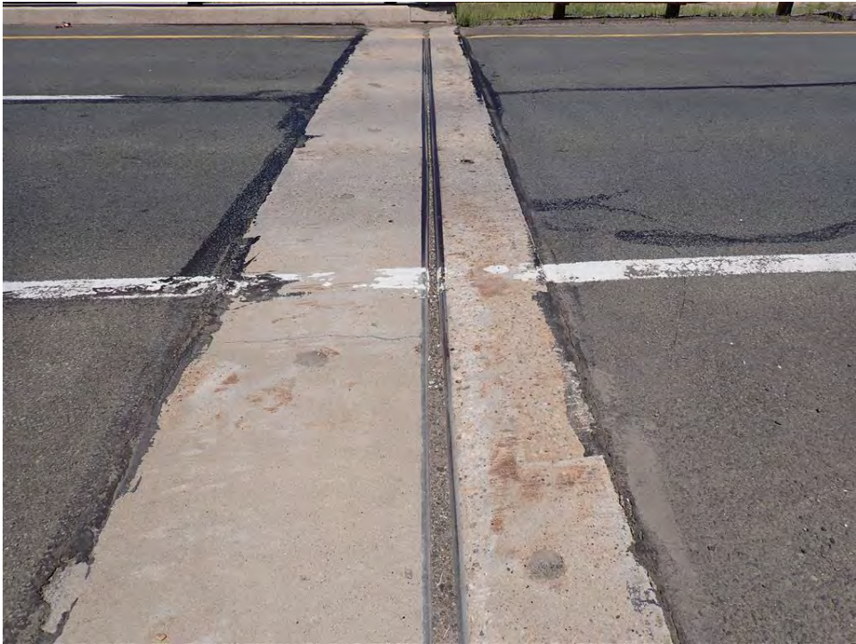
Photo 24: Dirt in Expansion Joint at Bridge over US 287, Eastbound
