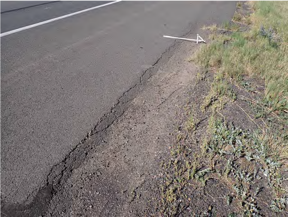
Photo 6: Rutting in North Shoulder, Westbound Off-Ramp at US 287
