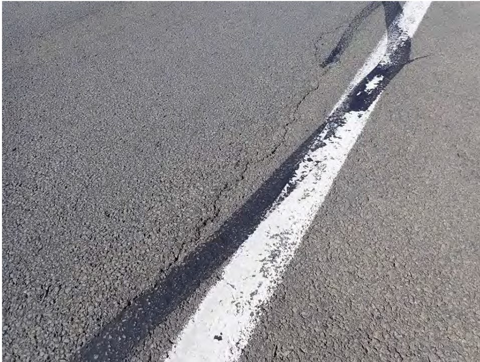
Photo 12: Poorly Sealed Longitudinal Crack in Asphalt, Westbound at Milepost 48.7
