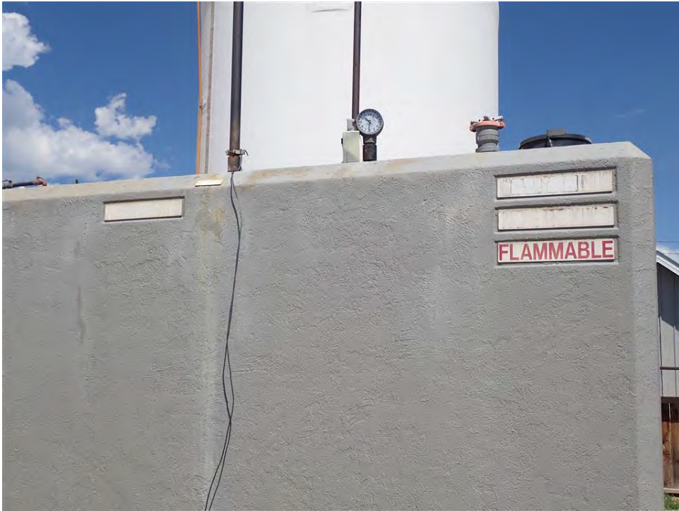
Photo 70: Faded Signs on South Side of Diesel Fuel Tank
