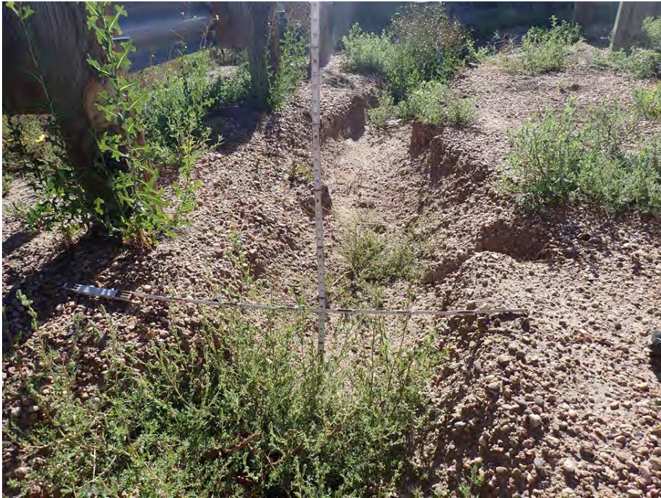
Photo 32: Erosion Trough in Median, Milepost 46.95
