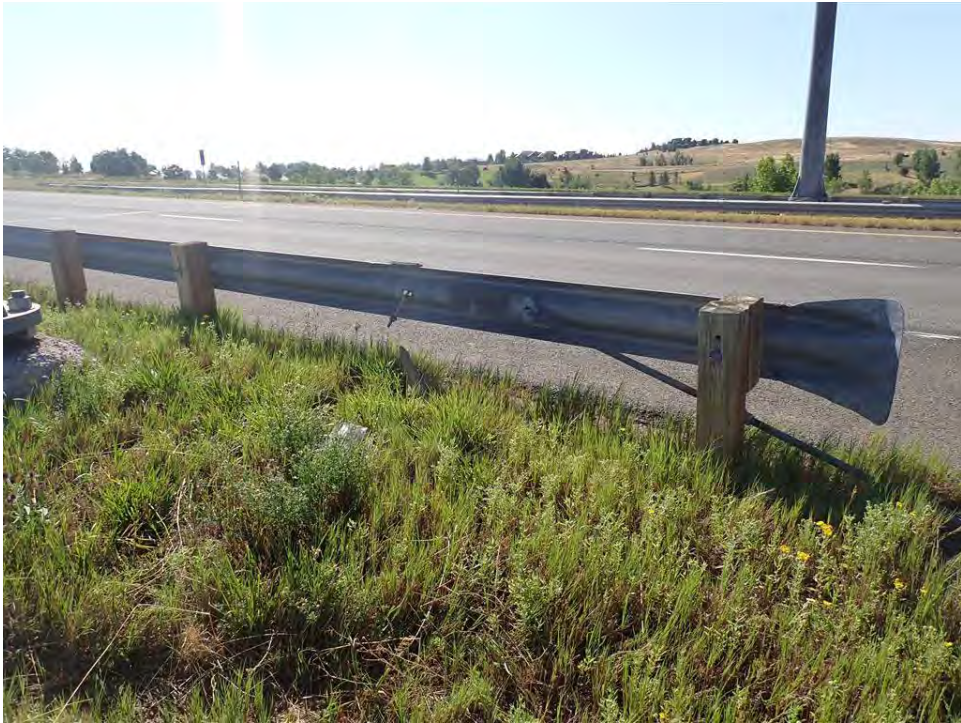
Photo 48: Damaged Guardrail Post, Westbound at Milepost 48.75
