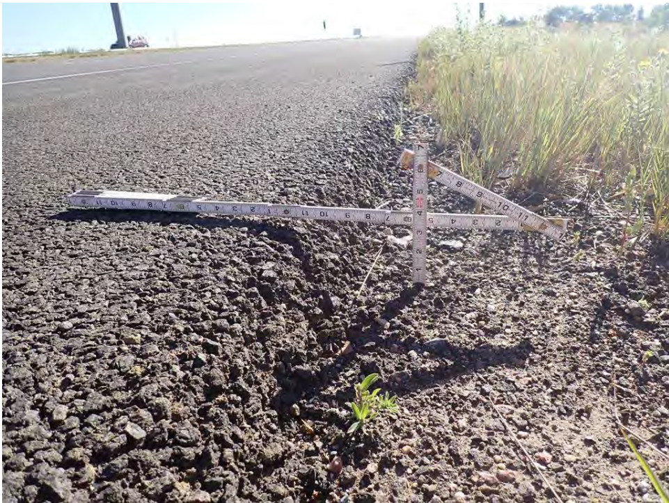
Photo 30: Shoulder Drop-Off, Eastbound at Milepost 48.75
