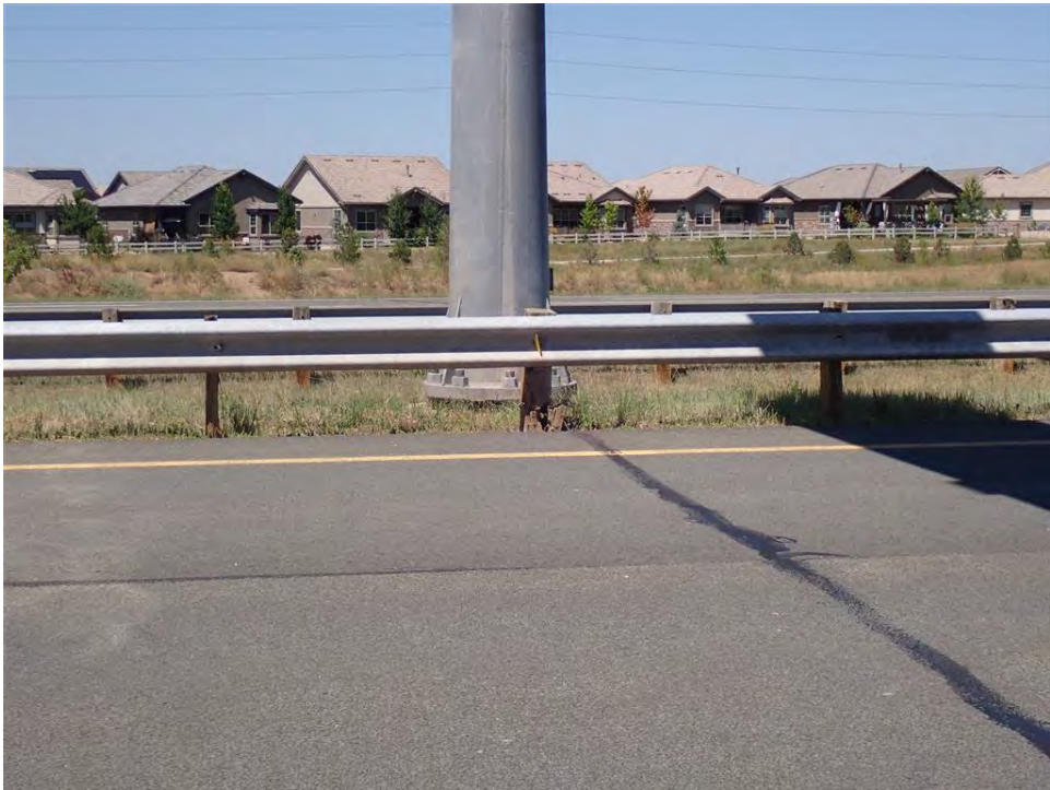
Photo 50: Typical Missing Timber Blockings in Median Guardrail (Milepost 51.05 Pictured)
