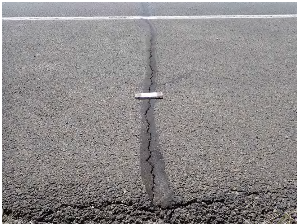
Photo 10: Previously Sealed Transverse Crack in Asphalt Re-cracking, Westbound at Milepost 53.3
