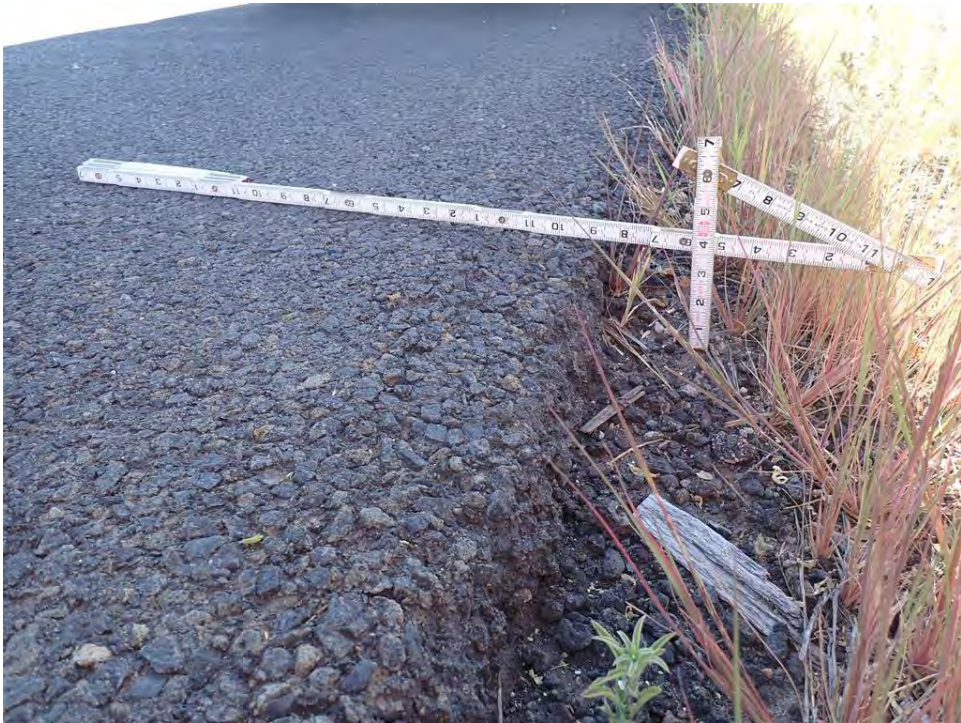
Photo 30: Shoulder Drop-Off, Eastbound at Milepost 48.75
