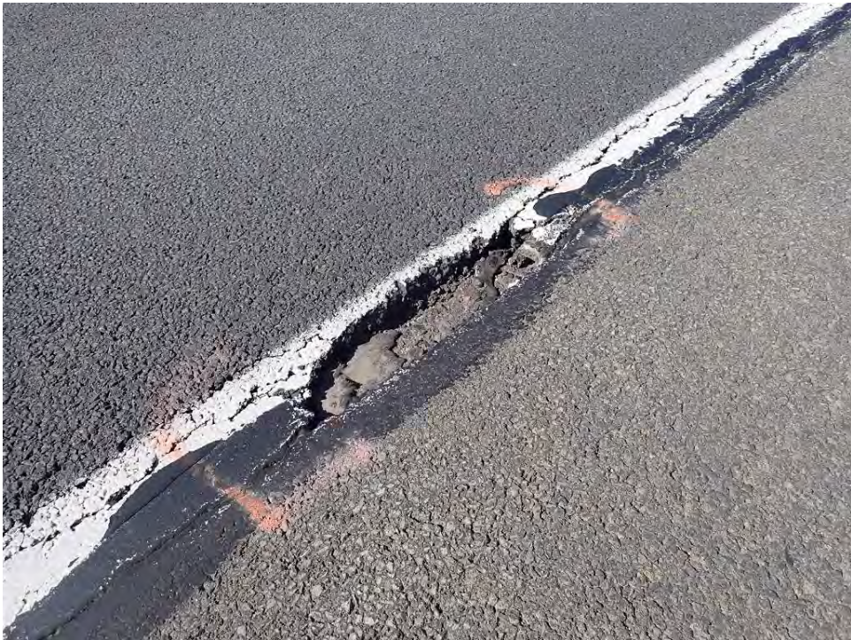
Photo 14: Patched Pothole in Asphalt, Westbound at Milepost 48.15
