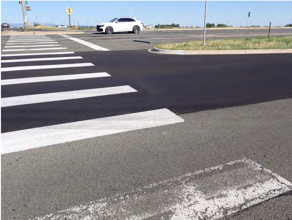
Photo 16: Repaired Potholes in Asphalt, Eastbound at 96 th Steet
