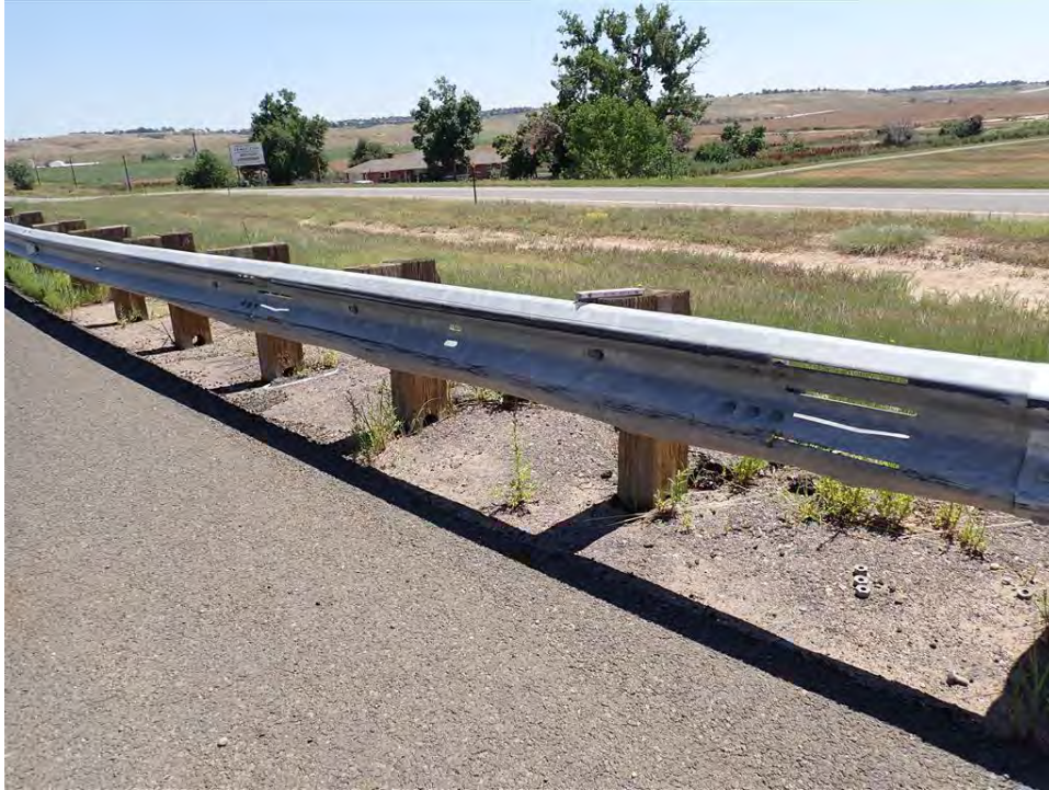
Photo 52: Impact Damage to Left Curb, Westbound at Milepost 52.15
