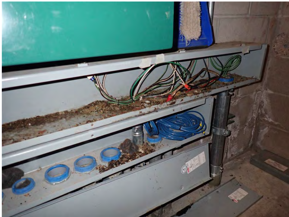
Photo 62: Evidence of Mice in Electrical Cabinet in Toll Booth Building, Westbound On-Ramp at US 287
