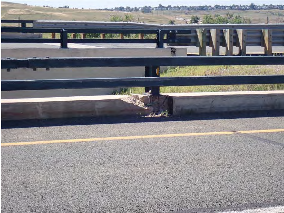
Photo 52: Impact Damage to Left Curb, Westbound at Milepost 52.15
