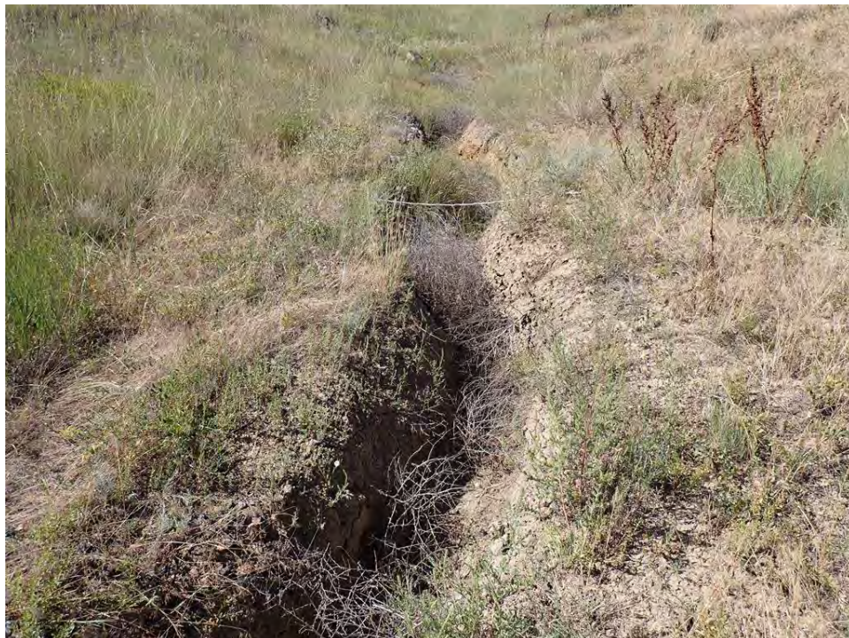
Photo 34: Erosion Trough and Displaced Riprap in North Slope, Westbound at Milepost 51.05
