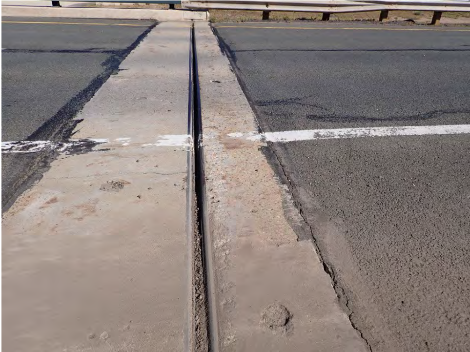
Photo 26: Shoulder Drop-Off, Eastbound at Milepost 51.15
