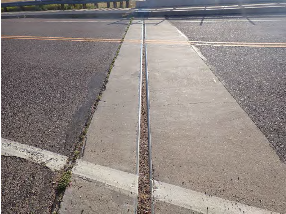
Photo 22: Dirt in Shoulder of Expansion Joint at Bridge over Eastbound Dillon Road, Westbound
