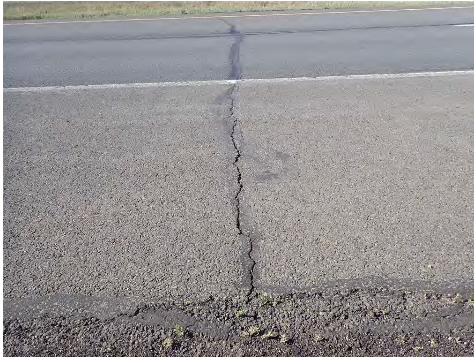
Photo 10: Previously Sealed Transverse Crack in Asphalt Re-cracking, Westbound at Milepost 53.3
